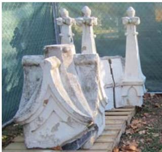
Crumbling stonework is being removed and will be sent to a foundry where molds will be made. The molds can then be used to cast replacement pieces.
