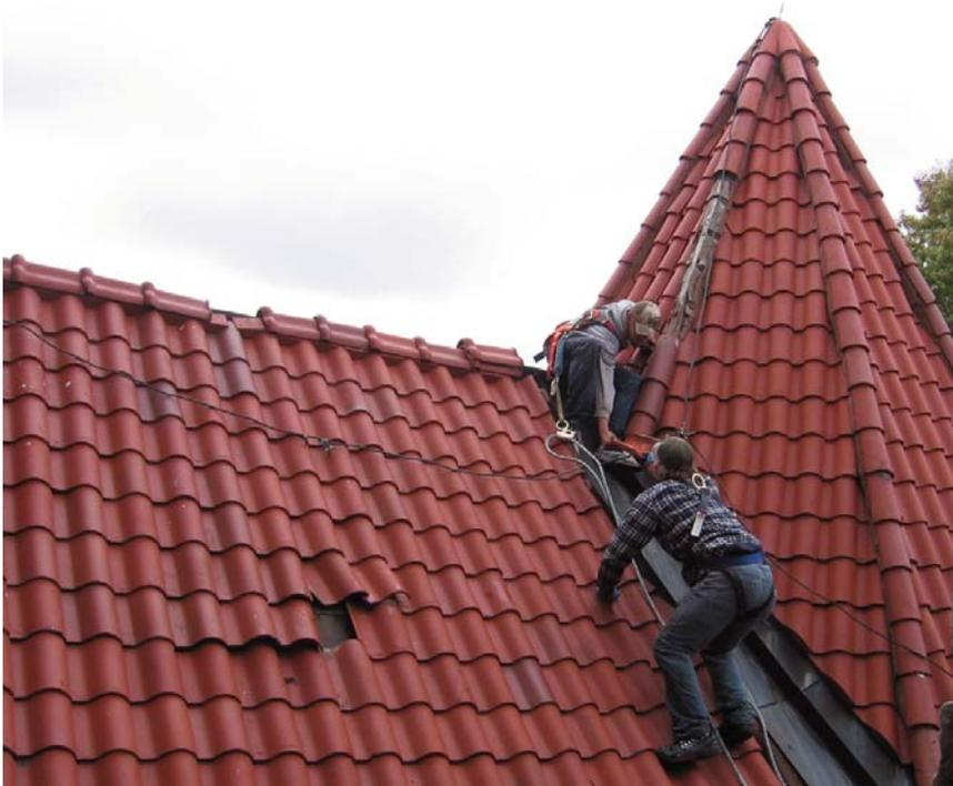
The church's tile roof receives repair work from the Pro Tech crew. Work was done to the cupola tower above the parlor and other parts of the wide tile roof areas.
